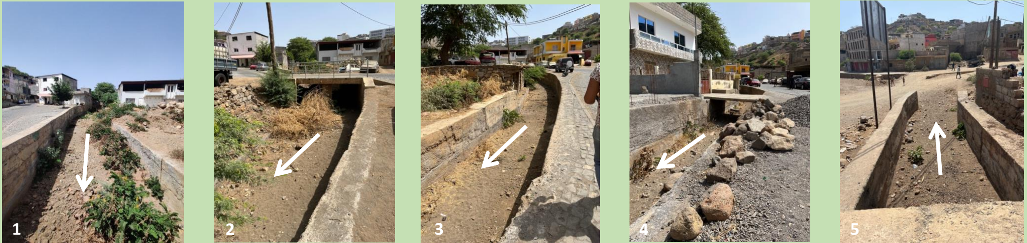
Figure 20 Pictures of observation marks drainage channel B. (Source: A. Sayyad-Hartounian)
