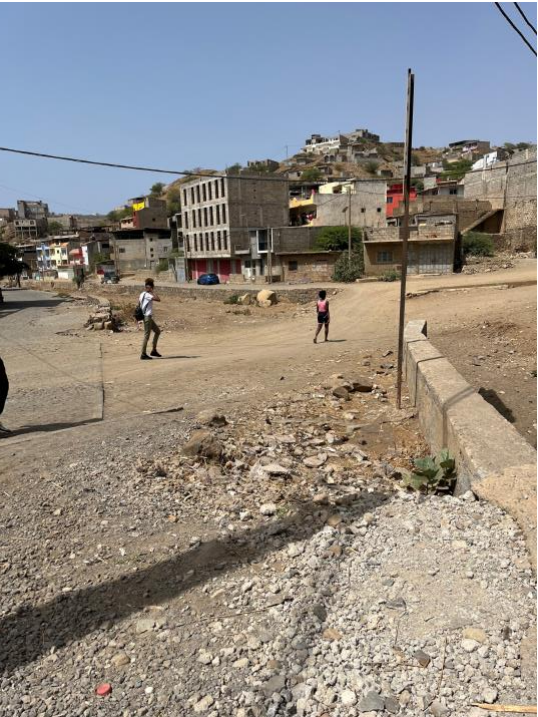
Figure 17 Unpaved road blocking drainage channels A & B and the mainstream of the Safende river. (Source: A. Sayyad-Hartounian.)
