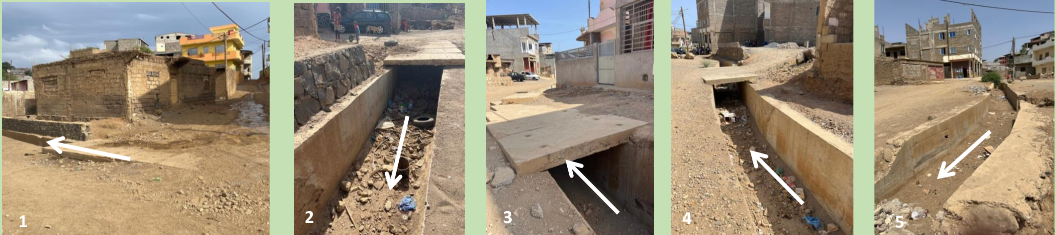
Figure 16 Pictures of observation marks drainage channel A. (Source: A. Sayyad-Hartounian).
